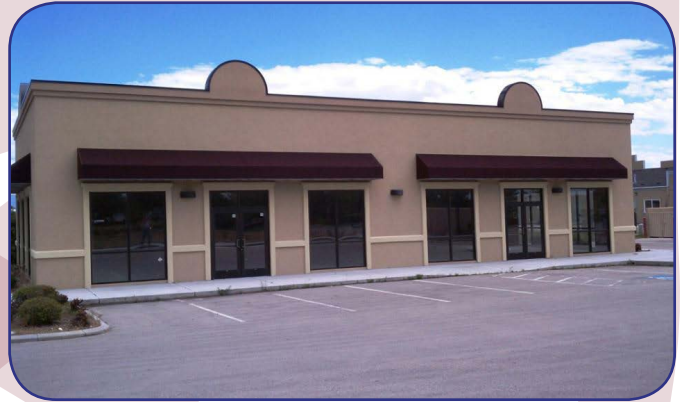
The new Star Baptist Church building.
